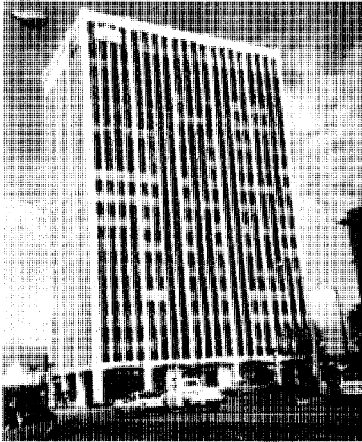
Above The Colorado Springs H&H office in Palmer Center.
