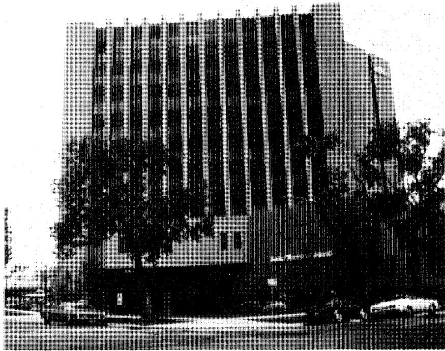
Right Office building for the H&H lawyers in Cheyenne, Wyoming.
